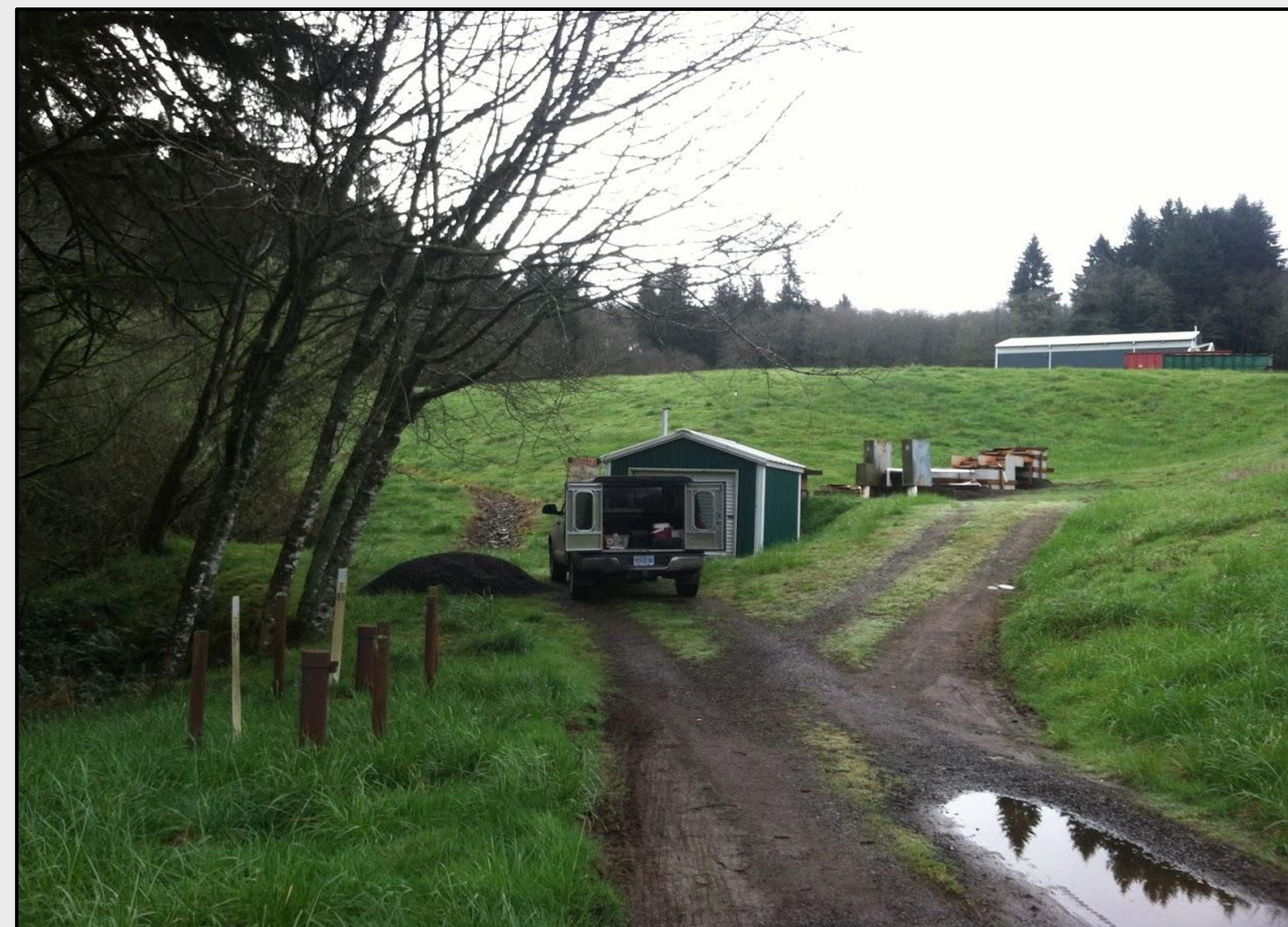
Figure 1. Site area available for a leachate treatment system at the landfill.
