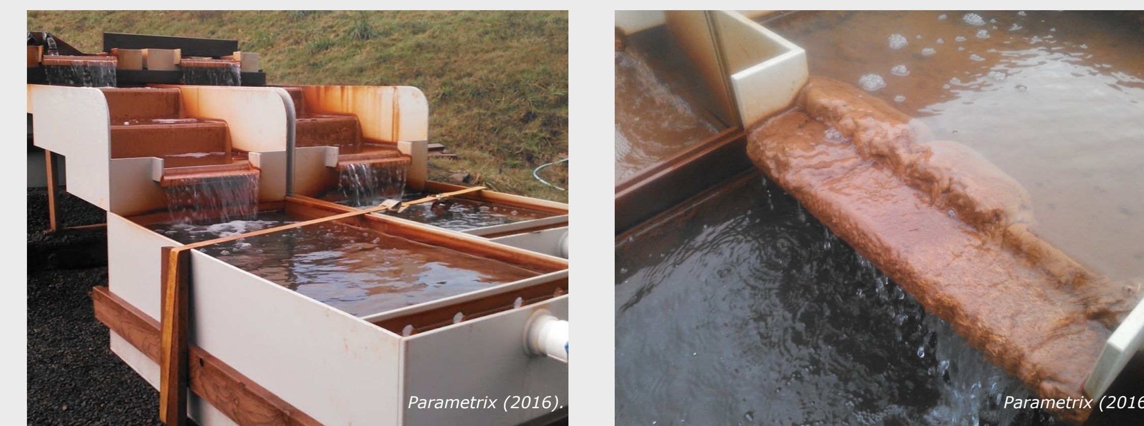
Image 3. Parametrix pilot study of cascade aeration, polymer flocculation, and settling experienced excess clogging and build-up from the iron precipitate.
