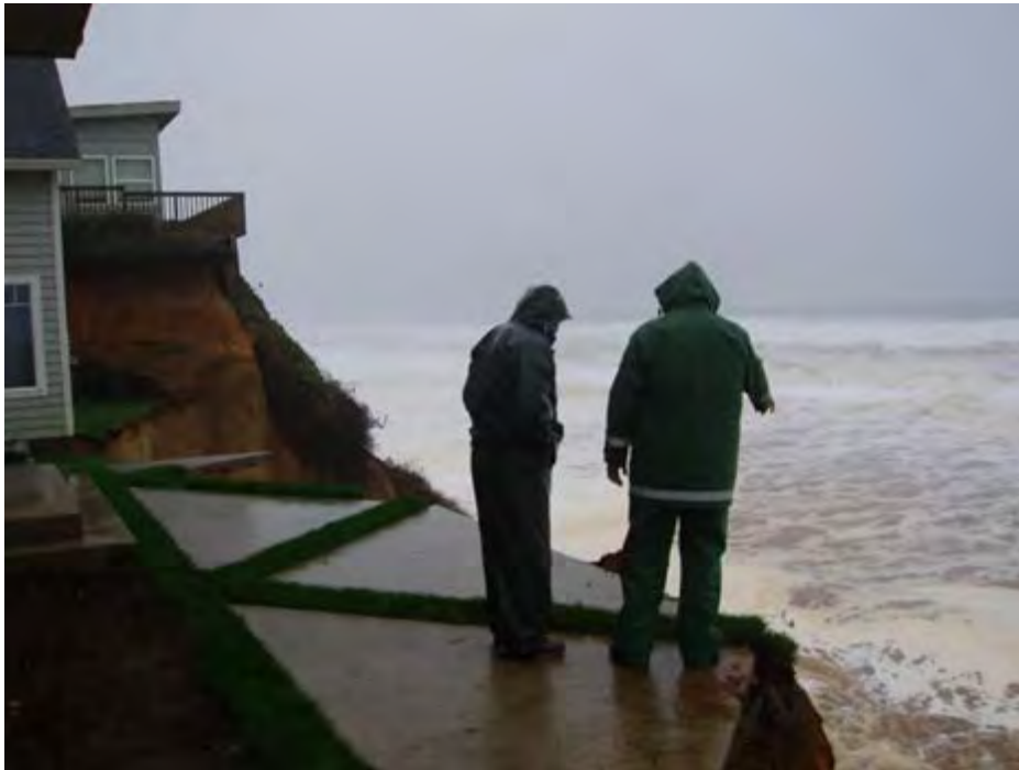
Figure 55. Bluff Failure Due to Toe Erosion by Ocean Waves
