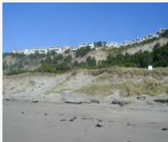
Figure 54. Erosion at “The Capes” Condominiums, Oceanside, Oregon
