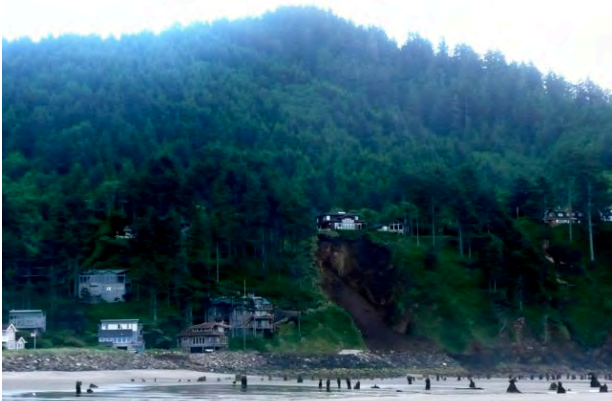
Figure 83. Landslide in Tillamook County
