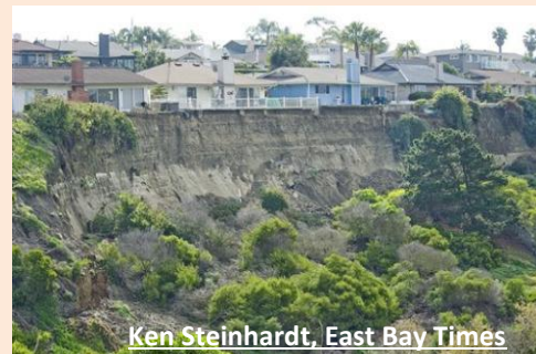
2011 Landslide in Contra Costa County
