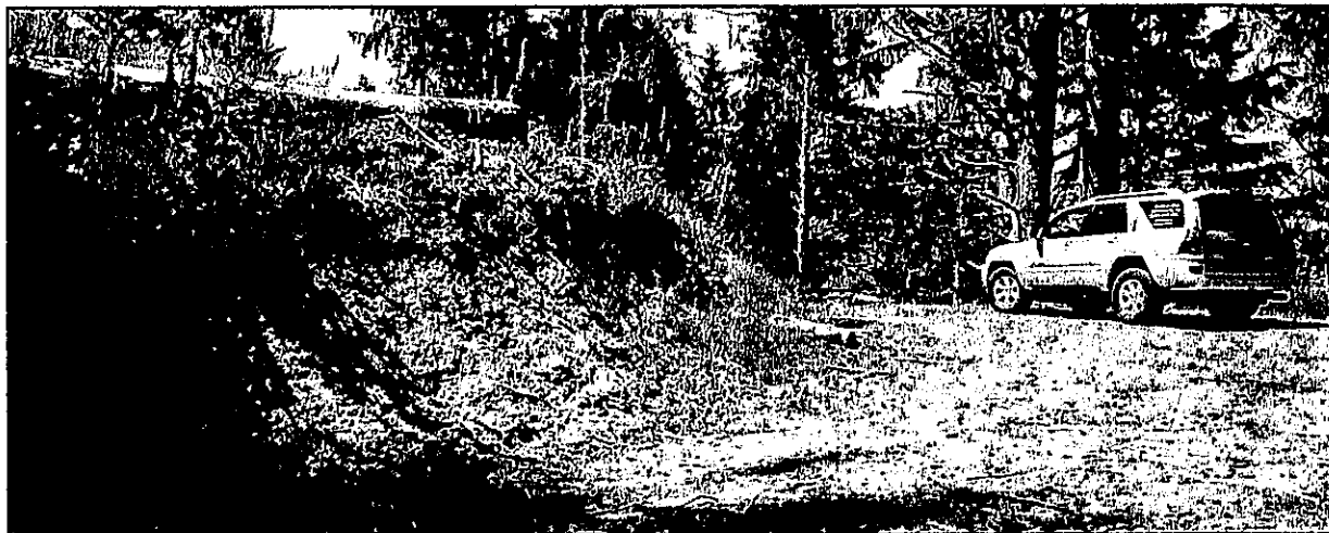
Photo 1 – Existing cut slope on southern margin of driveway, adjacent to home site on upper elevation of Tax Lot 500. The view is to west-southwest from near the west end of the existing driveway.
