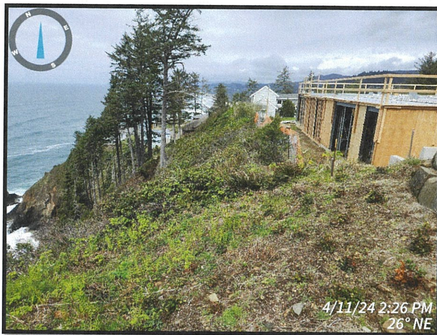
Photo 2: Recent conditions of the subject property, viewed from southwest looking north-northeast.
