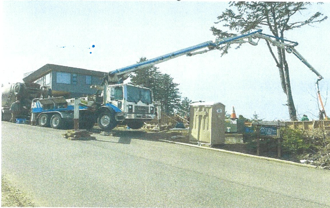
View of the tree from road trunk lean, limb dieback, crown top heavy.
