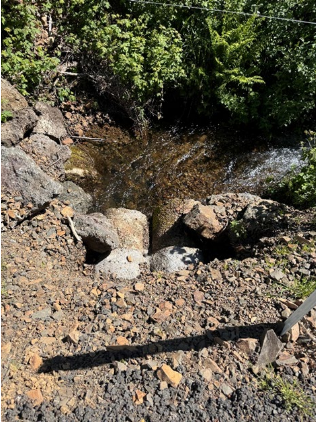
Figure 4: Inlet from top of road
