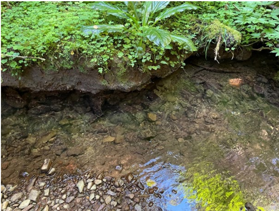
Figure 6: Substrate upstream from culvert
